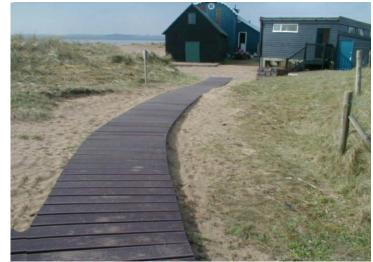
explains, is that with KC-Deck being 48mm thick only two supporting stringers were needed, whilst with more flimsy material extra cost would have been involved in buying and installing three stringers. He also felt that the colour and the non-slip surface more appropriate over the sand -dune terrain.
